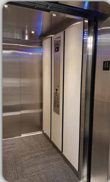
Brushed Stainless Steel car with custom laminate panels
